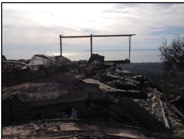
Hot Springs Lane - PDU destroyed
