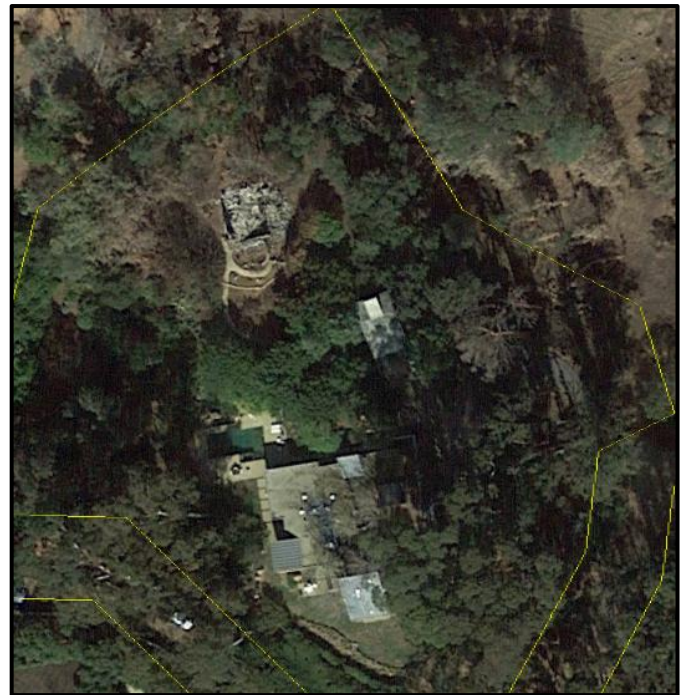
East Mountain Drive - post-Thomas Fire (Source: Google Earth)
