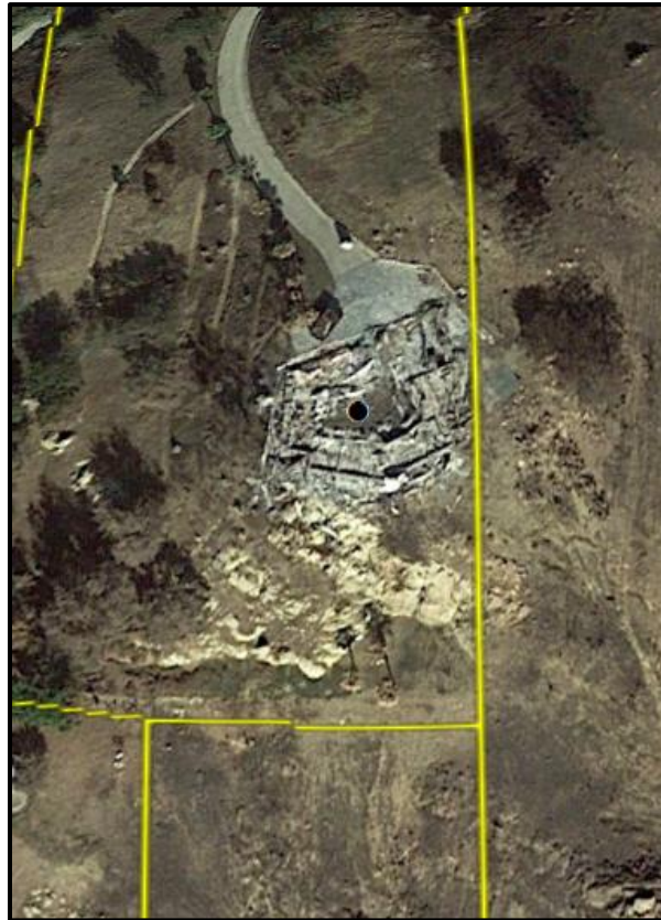
Hot Springs Lane - post-Thomas Fire (Source: Google Earth)
