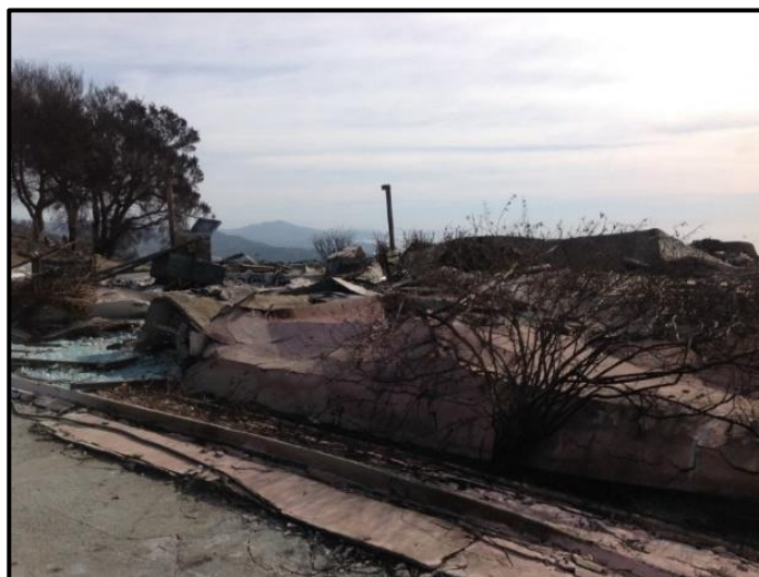
Hot Springs Lane - PDU destroyed
