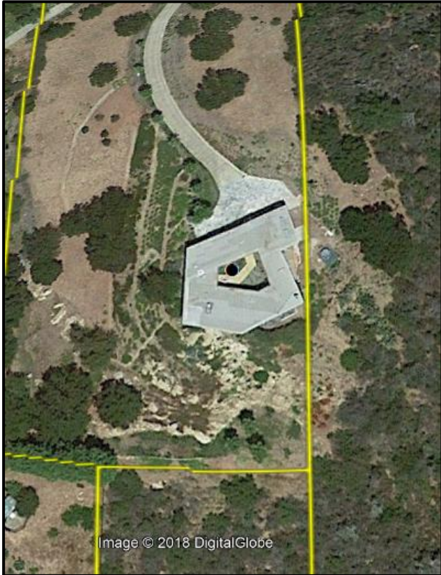
Hot Springs Lane - pre-Thomas Fire (Source: Google Earth)
