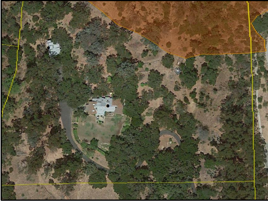
East Mountain Drive – pre -Thomas Fire (Source: Google Earth)
